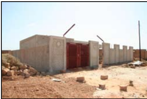
Niamey house under construction.
